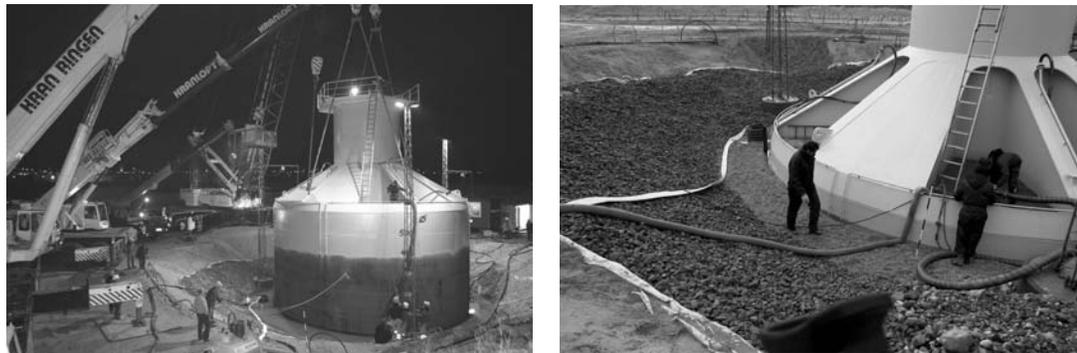
Figure 3 Installation of the prototype foundation at the test site in Frederikshavn, a) during installation and b) after installation.
